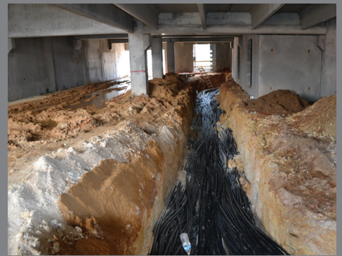
Through parking garage for new apartment complex.
