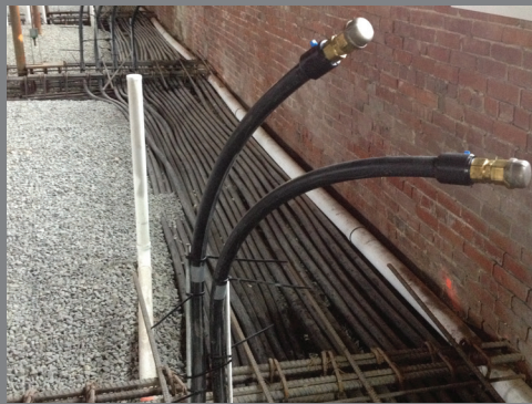
The flexibility and long lengths of TracPipe PS-II allowed for a total install time of just 36 hours versus an estimated 1200 hours for black iron pipe.
