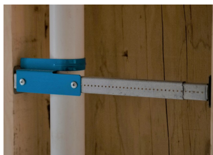
Overhead pipe installation in-between joists and beams
