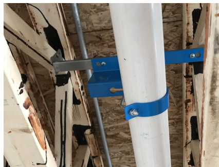
Overhead pipe installation in-between joists and beams
