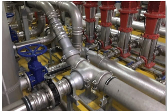
GroovJoint fittings installed
